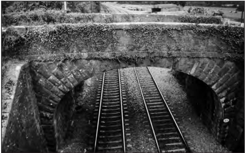
The railway bridge at Stacumney before demolition and replacement in 2007.
